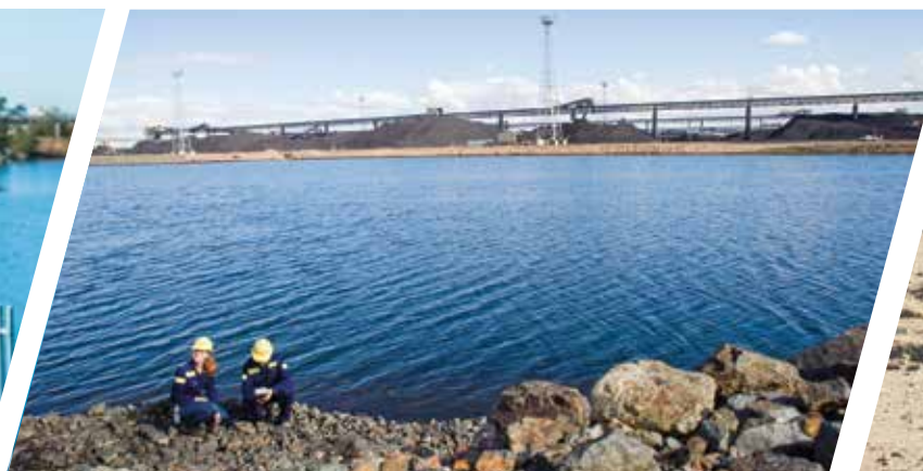
Monitoring of discharge ponds ensures GPC is compliant with environmental obligations (above and at right)
