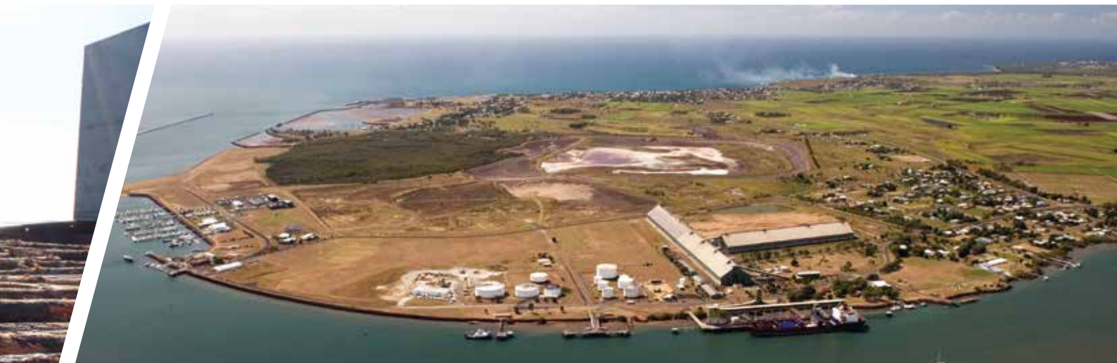
GPC's focus in the short to medium term is to increase the use of existing port infrastructure at the Port of Bundaberg
