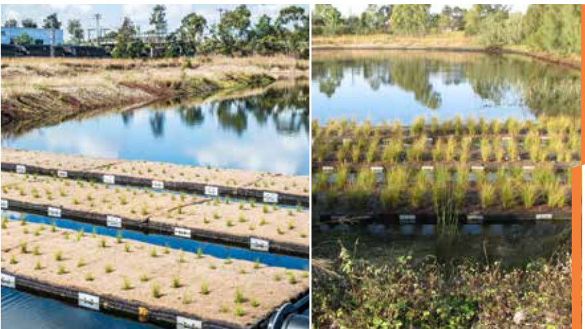
This floating wetland, planted more than 12 months ago (far left) is made from expanded polypropylene mats, and covered with coconut matting with pockets for suitable tube stock plants to grow in (right shows 12 months growth)
