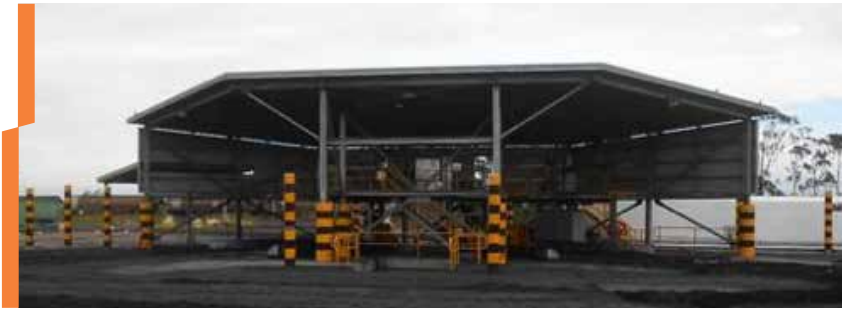
A new dual fuel bay was installed this year at RGTCT
