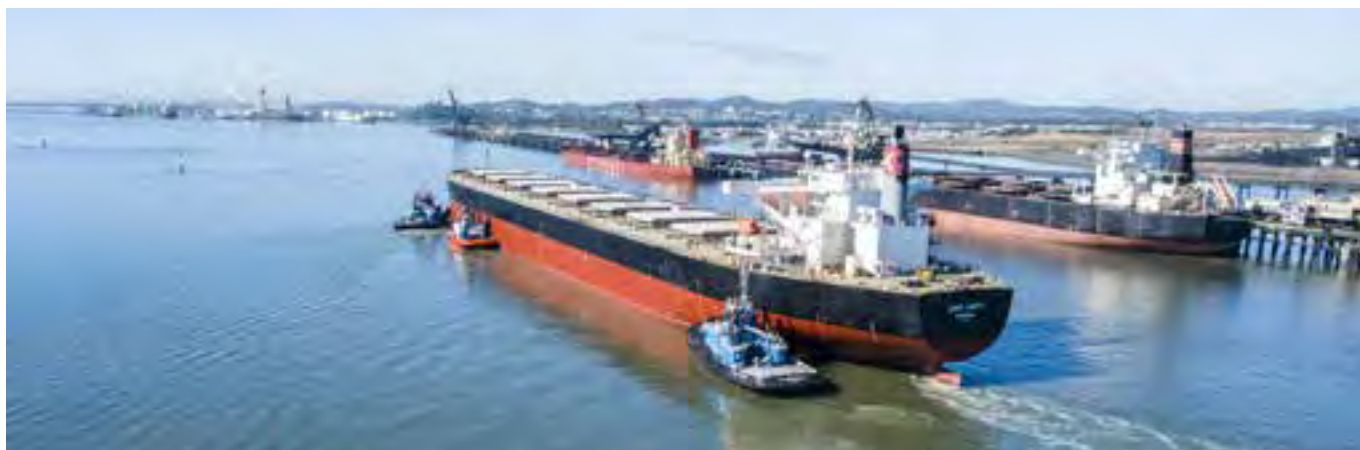
The widening of the Clinton Channel will provide a long-term solution and provide a safer passage for increasing Capesize vessel traffic
