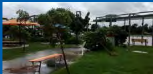
The East Shores precinct suffered significant damage at the hands of Cyclone Debbie, just hours prior to a major cruise ship market. Parks and Recreation teams worked around the clock to reopen the popular facility
