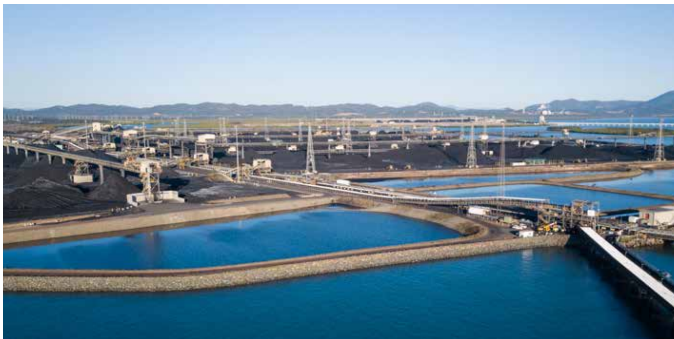
The long-term management of our structural assets has been a key initiative.
