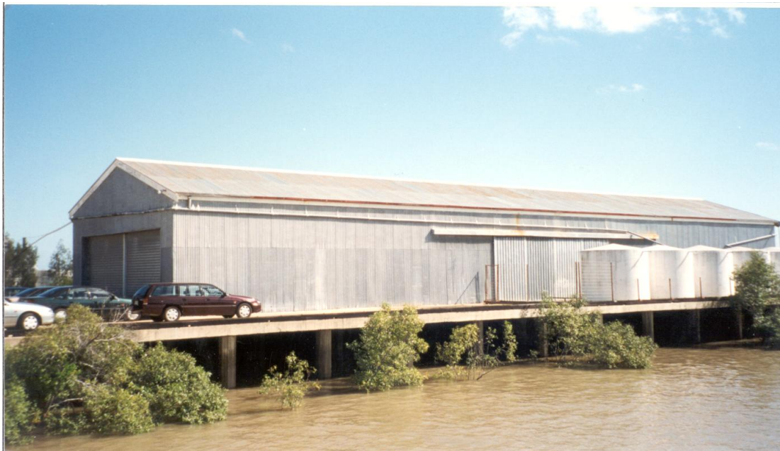
The Bulk Store No.1 viewed from the amenities building (south east).
