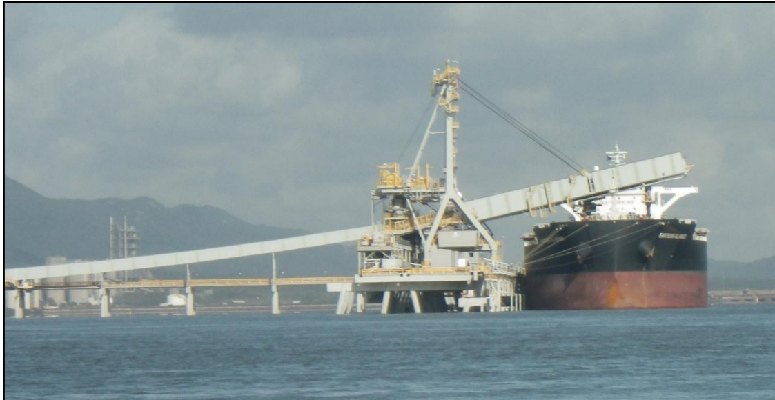
Figure 1-2 The Wiggins Island Coal Export Terminal (WICET), February 2017
