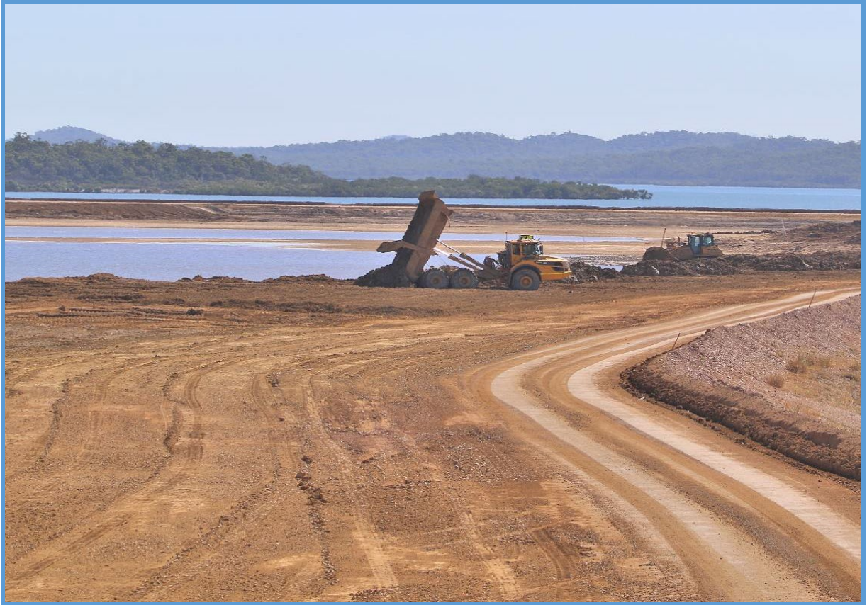
Figure 5: Placement of dredge material in the Reclamation Area
