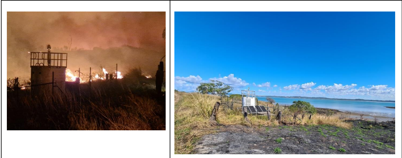
FIGURE 9. GPC LEAD LIGHT ASSETS GPC leadlight shown during and post burn
