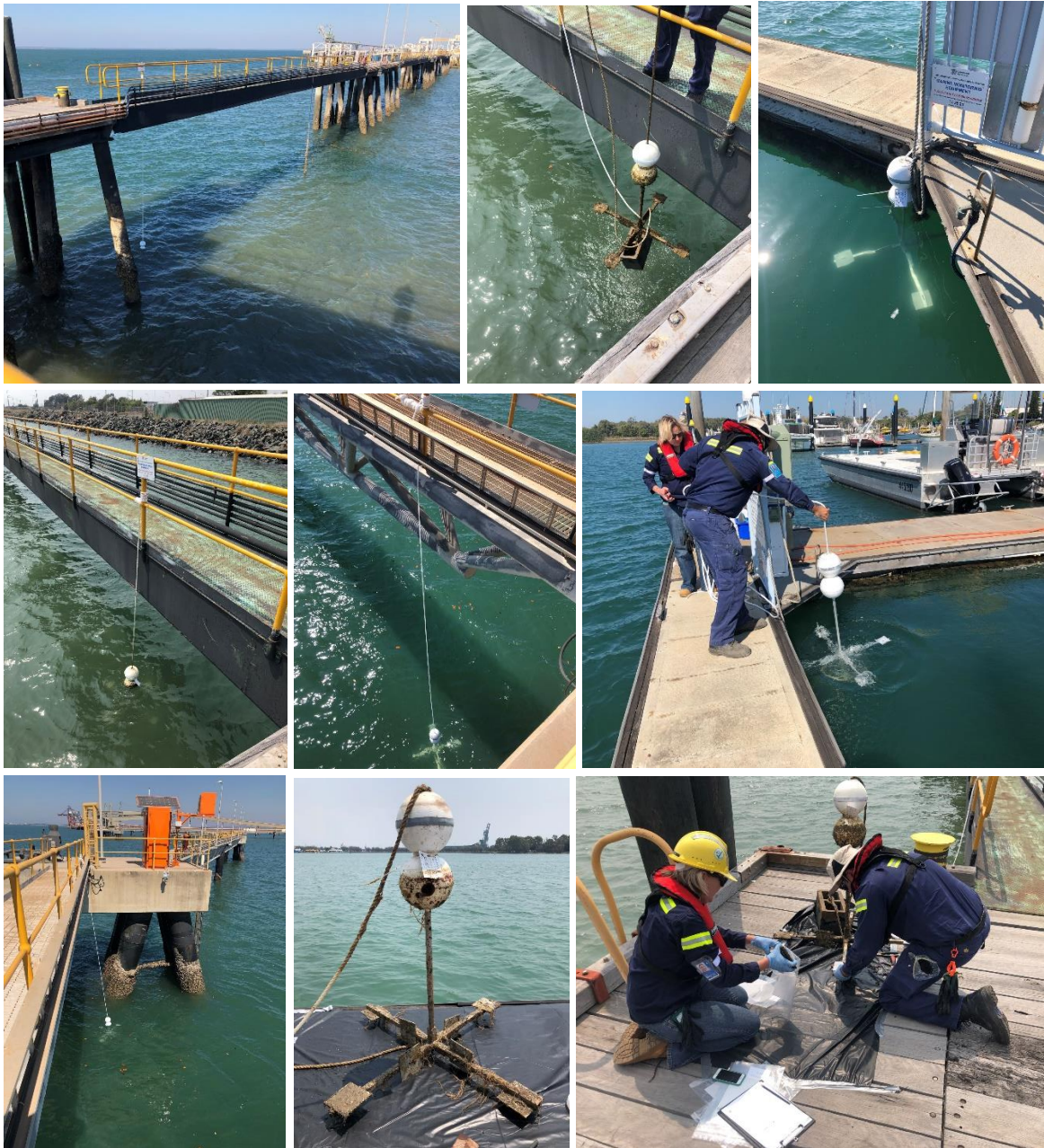
Figure 6: Settlement array deployments and retrievals at the Port of Gladstone
