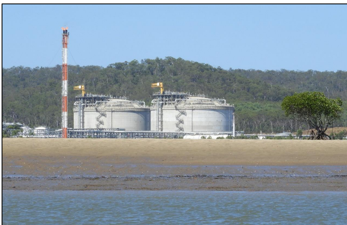
Figure 1-1 LNG plant on Curtis Island, February 2018
