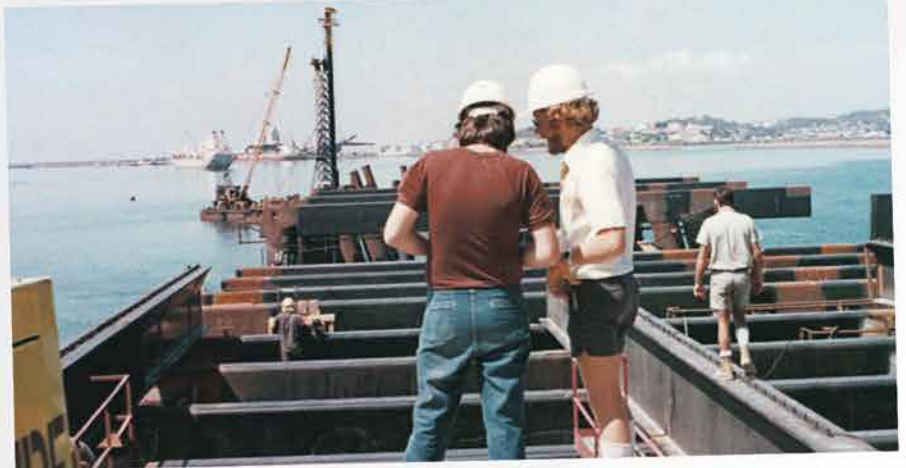
ABOVE: Construction commenced for Stage 2 of the Clinton Coal facility.
