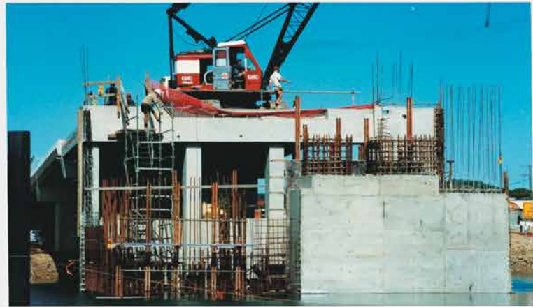
ABOVE: Construction of the bascule bridge across Auckland Inlet progresses.
