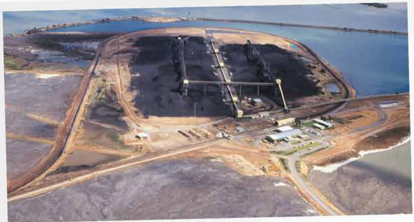
ABOVE: Additional stockpile storage progresses at the Clinton Coal Terminal.
