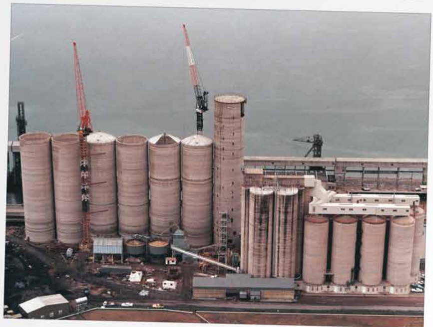
ABOVE: Six additional grain silos are constructed at Auckland Point.
