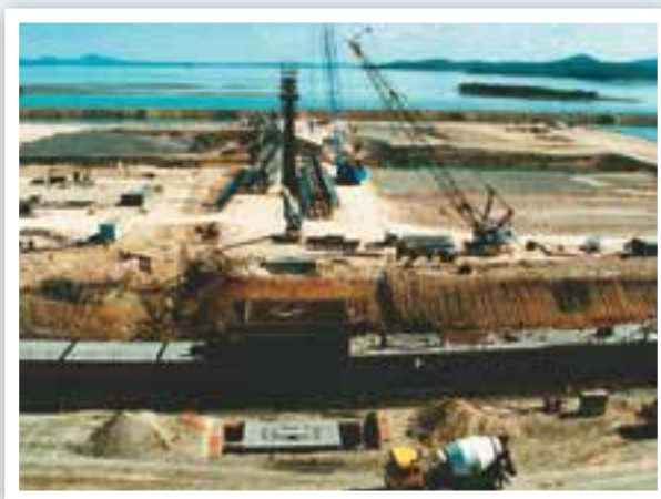
Stockpile 13 under construction at RGTCT.
