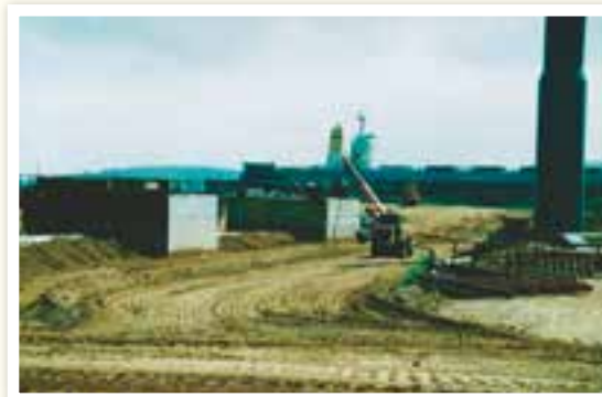
Construction commences on infrastructure for Stockpile 16 at RGCT, March 2003.
