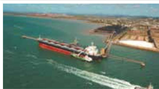
An upgrade of Barney Point's shiploading stream strengthened its capacity to 7mtpa.
