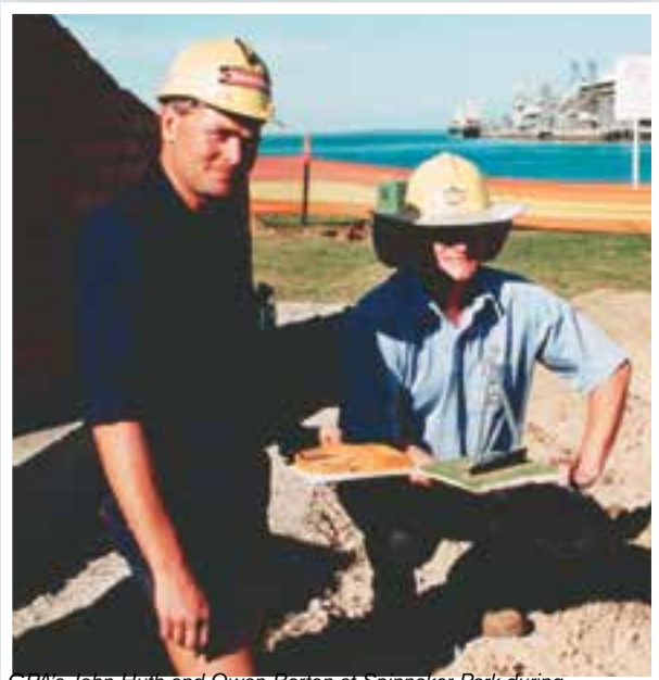
GPA's John Huith and Owen Barton at Spinnaker Park during its construction, July 2000.
