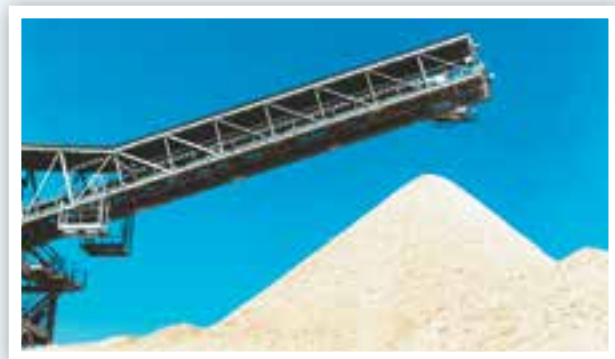
Calcite stockpile, Auckland Point.
