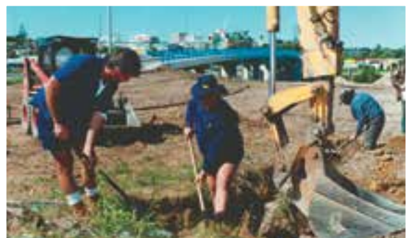
GPA employees undertake earthworks at Gladstone Marina, July 1997.
