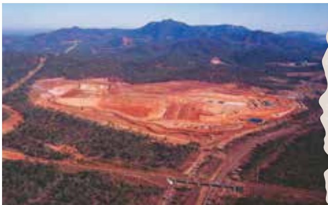
The Comalco Alumina Refinery under construction, June 2002.
