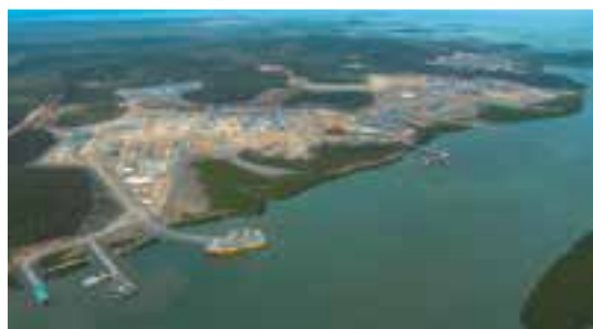
Construction of the three LNG plants on Curtis Island continued throughout 2012 – 2014.
