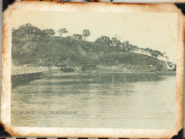
TOP: Auckland Point, 1923. Wharf under construction. ABOVE: Passengers from ship to train at Auckland Point Jetty, 1909. LEFT: Auckland Hill, ca 1920. Photo courtesy of Gladstone Regional Art Gallery and Museum.
