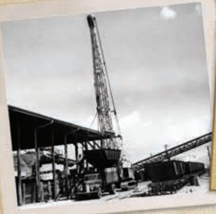
BELOW: Auckland Point 1954. Receiving hopper fed from conveyor to wharf.
