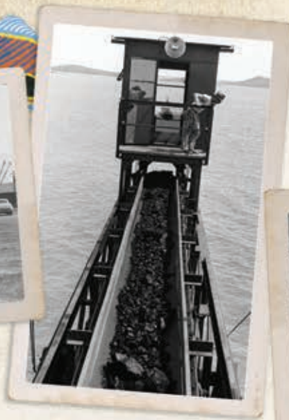
LEFT: Auckland Point 1954. Control cabin on end of fixed head loader.
