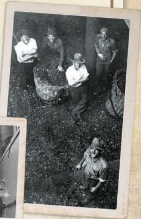
ABOVE LEFT TO RIGHT: (1) Auckland Point 1947. Loading coal into rail wagons. (2) Coal from the Callide Valley being loaded for overseas shipment onto the cargo ship Barossa. 1948. Image courtesy State Library of Qld. (3) Auckland Point 1950s. Tween decker vessel manual trimming carried out by shifting coal via cane baskets into corners of ship's hold.
