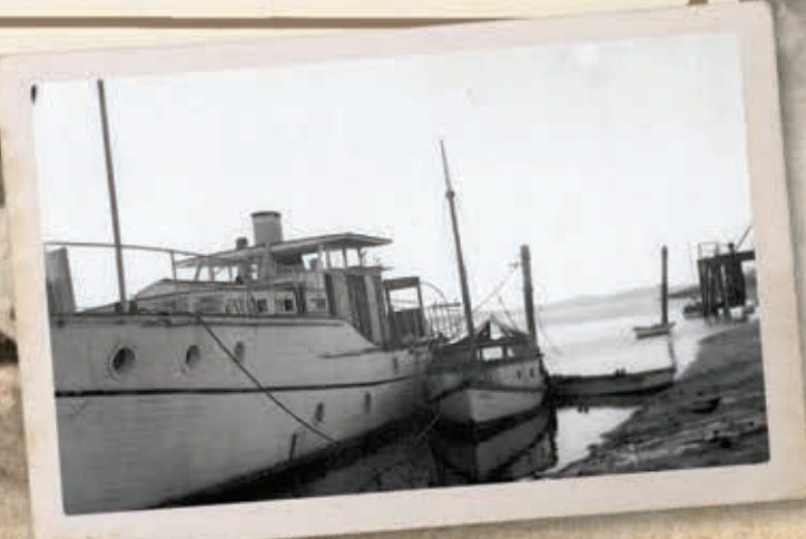
TOP TO BOTTOM: (1) Harbour and Garden Island from Ferris Hill. Circa 1930s. Image courtesy State Library of Qld. (2) Aerial of Gladstone Harbour. Circa 1938. (3) Serene weather at Auckland Creek. Circa 1930s. Image courtesy Jimmy Harris. (4) Low tide at Auckland Creek. Circa 1930s. Image courtesy Jimmy Harris. (5) Launch berthed at Auckland Creek. Circa 1930s. Image courtesy Jimmy Harris. MAIN BACKGROUND: Auckland Inlet and Goondoon Street 1952.
