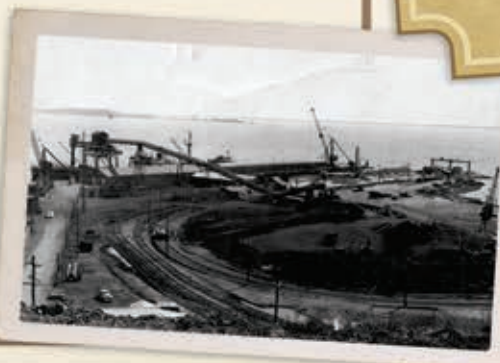
LEFT: Coal stockpiles at Auckland Point Wharf. 1954. Image courtesy State Library of Qld.
