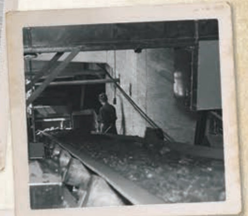
BELOW: (1) Auckland Point 1954. Coal loaded with new conveyor system. (2) December 1954. First coal loading (3) Auckland Point 1954. Mechanical bulk handling.
