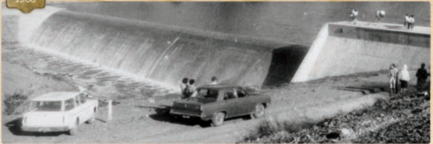
Asweya Weir overflows. Photo courtesy of Queensland Alumina Limited.
