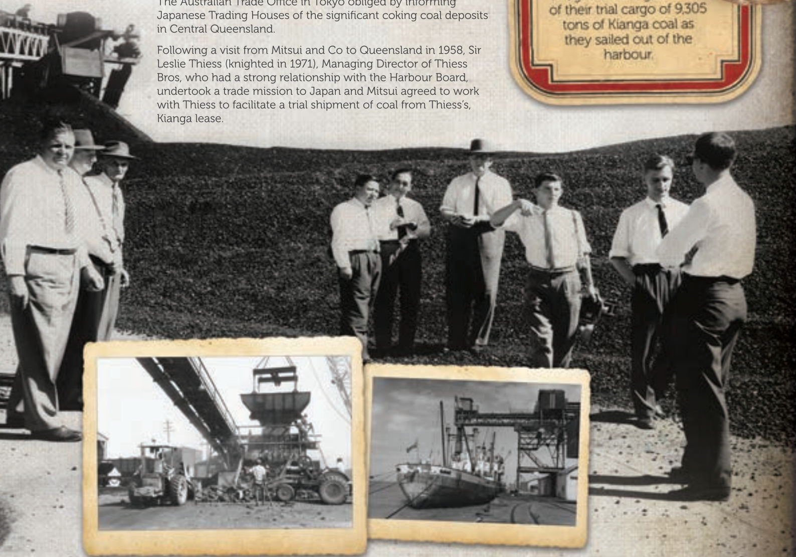
MAIN ABOVE: BELOW: December 1960 – Auckland Point Terminal laying down a shipment of Kianga coal destined for Japan. M. Hanson, GHB Deputy Chairman, J. O'Malley, Mayor, J. Burrows, State MLA for Port Curtis, E. Evans, Minister of Mining, Mitsui and Peabody personnel.
