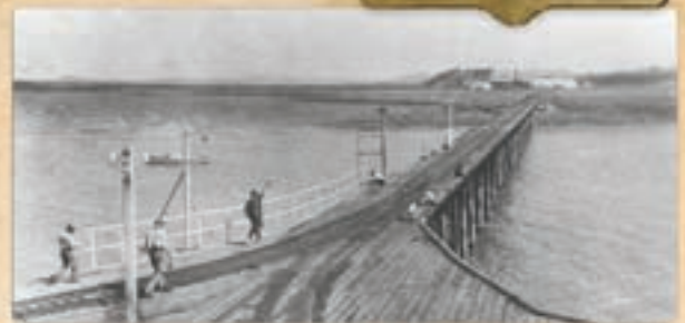
The meatworks jetty, now QM wharf. Photo courtesy of Gladstone Regional Art Gallery and Museum.
