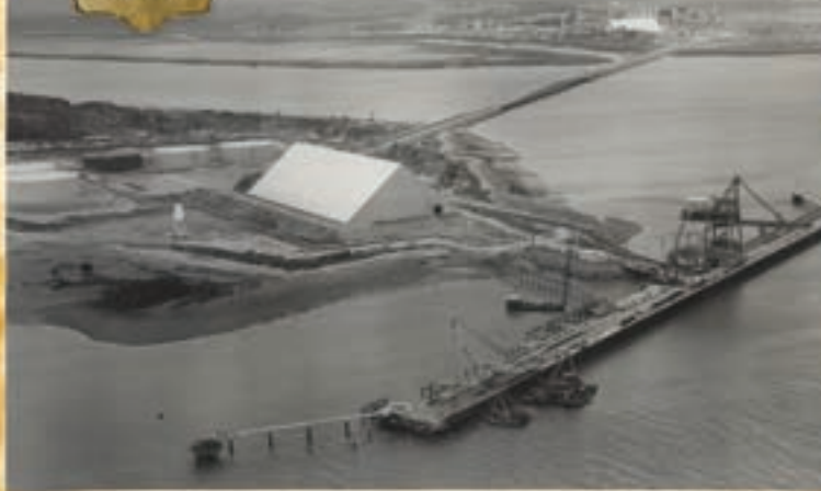
South Trees - Aerial - Wharf decking almost complete. Photo courtesy of Queensland Alumina Limited.
