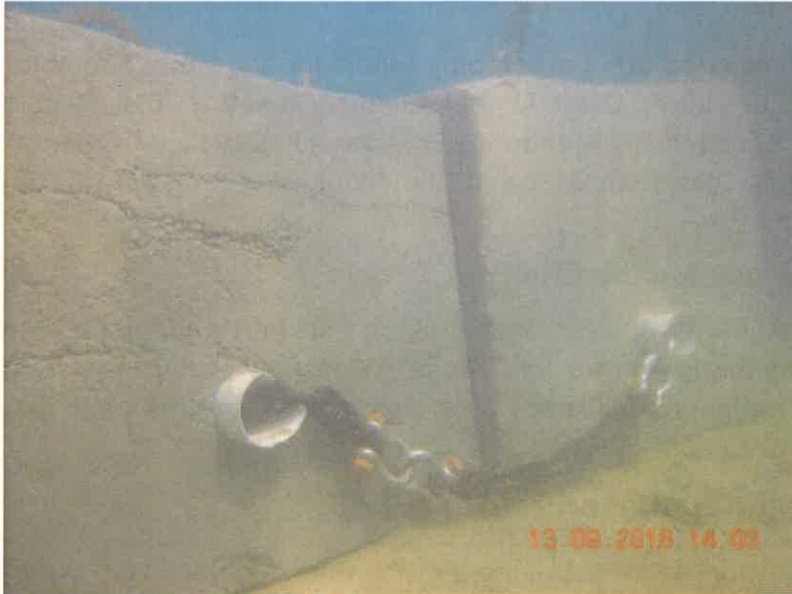
Figure 1: Mooring block in situ Pancake Creek.
