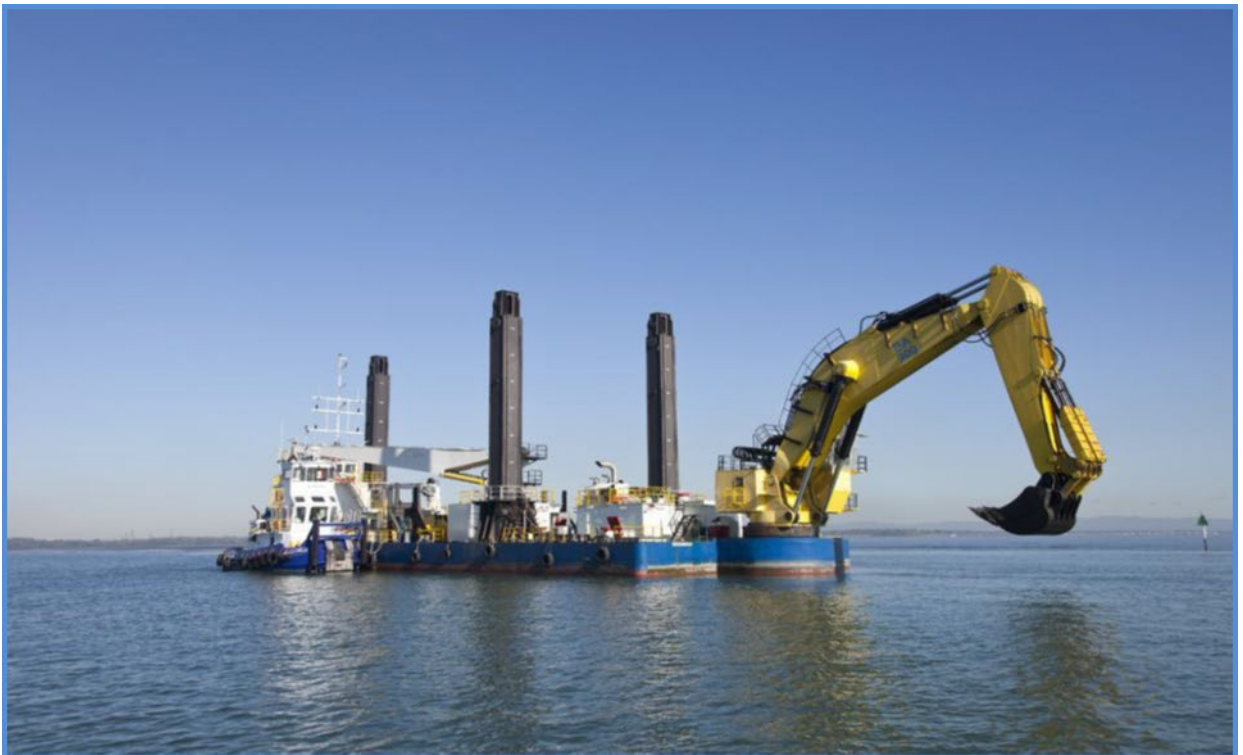
Cover photo: Back Hoe Dredge Woomera
