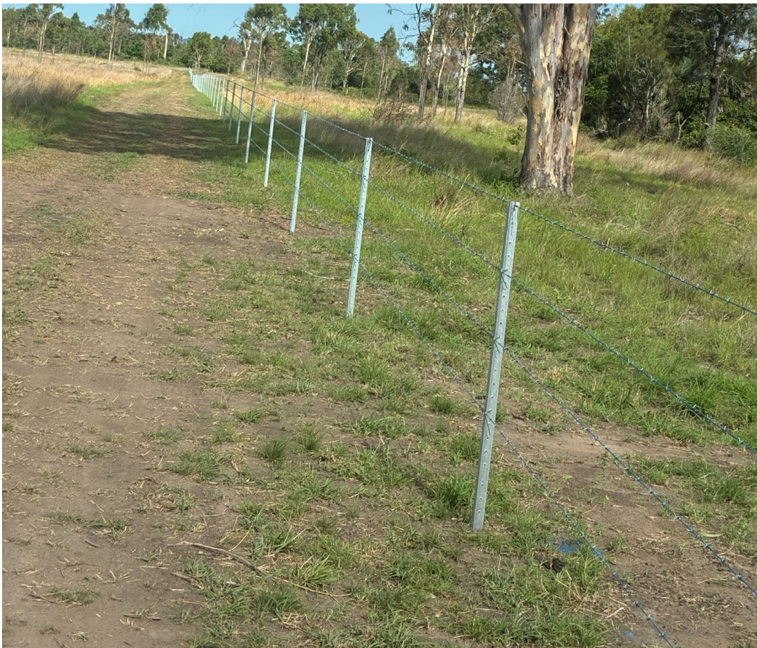
Image 4. Section of completed fencing (image captured December 2025)
