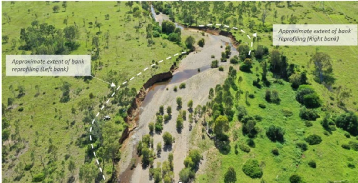
Image 1: Aerial imagery of the sites before construction commenced.
