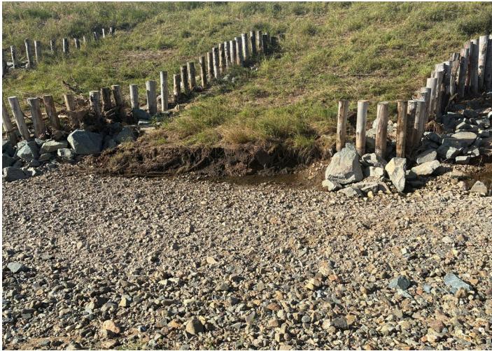
Image set 12. At Site Two, erosion affecting the second pile field following a high-flow event. Photographs taken on 23 March.
