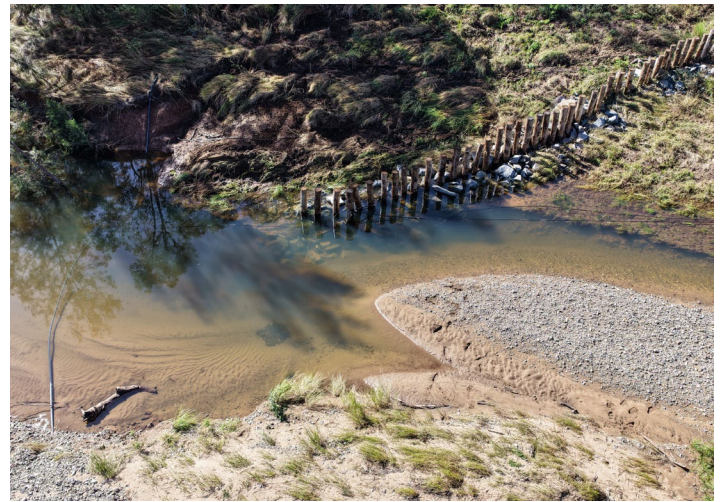
Image set 12. At Site Two, erosion affecting the second pile field following a high-flow event. Photographs taken on 23 March.
