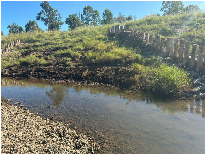
Image set 13. Pile Field One Left: Channel deepening at Site One (recovering)
