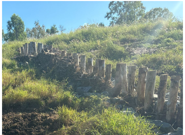
Right: Debris accumulation on the pile fields
