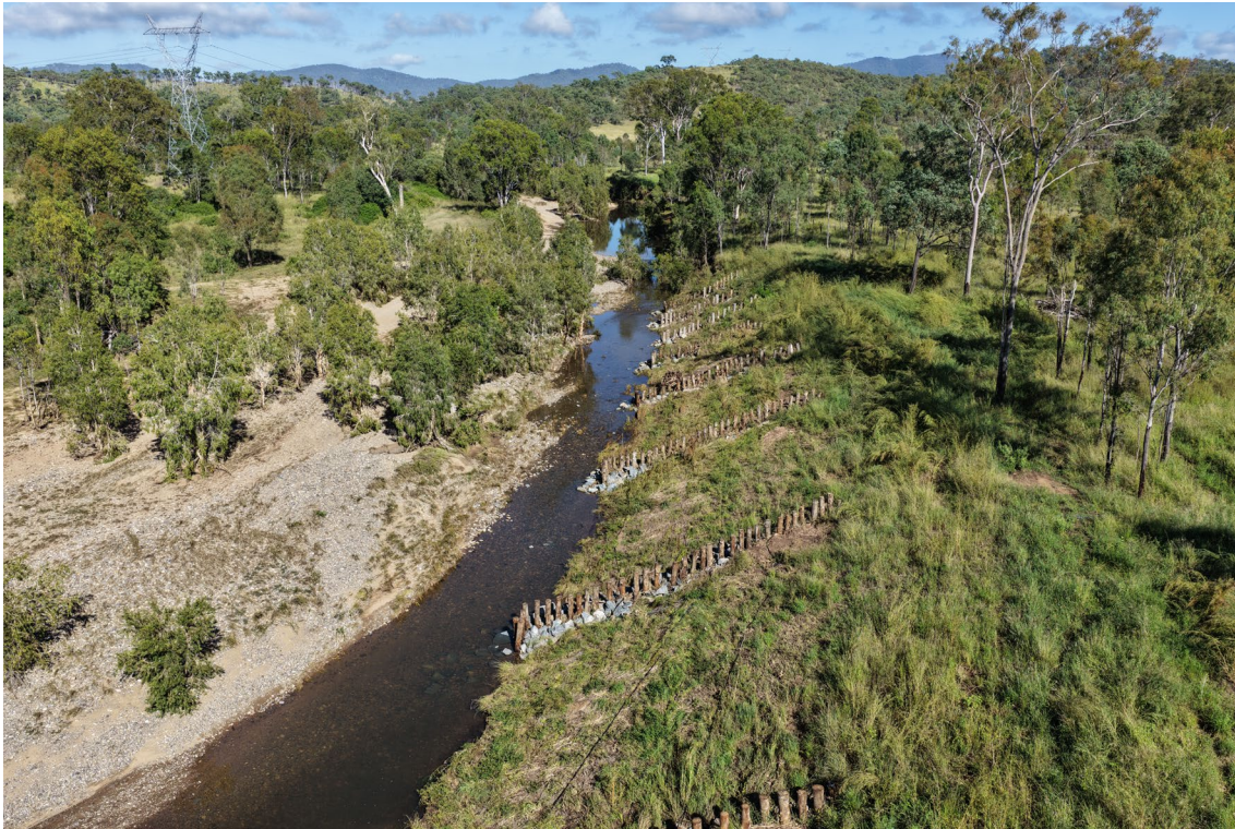
Image 2: Site 1 looking upstream (image captured 12 March 2026)
