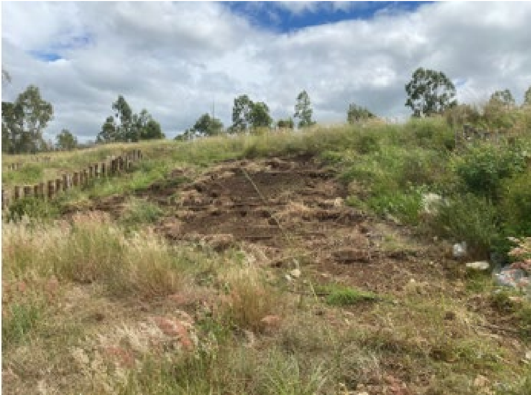
Image 11: Evidence of pig damage at Site One. Photograph taken on 23 March 2026
