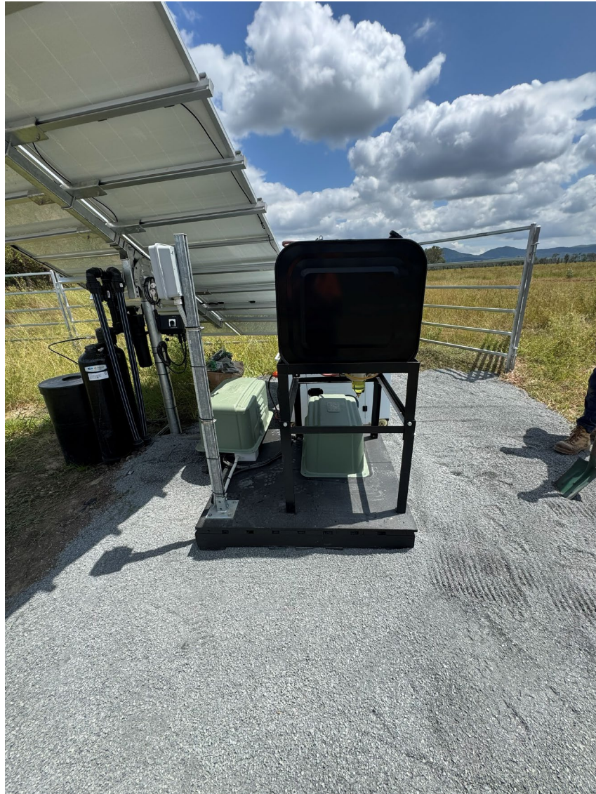
Image 6: Irrigation pump installation
