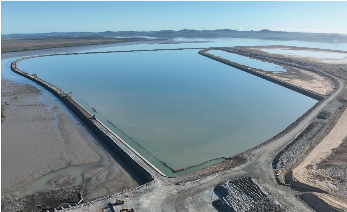
Figure 2: NLEP bund wall as of 2 September 2026
